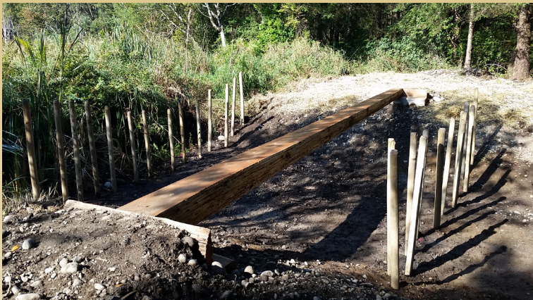
Beaver analogue, during construction.
