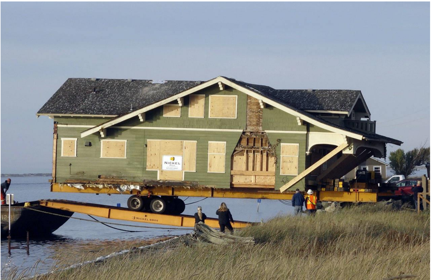
Crews from Nickel Bros. help unload a 1916 Sears kit house off a barge onto Cline Spit on Monday. Jim and Diane Luoma bought the house and moved it from Shelton. (Steve Jones)
