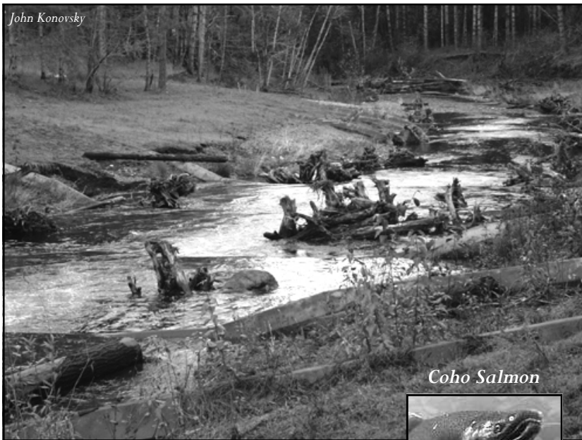
Goldsborough Creek approximately one year after dam removal. Concrete weirs control the grade of the stream channel, which salmon easily jump over.
